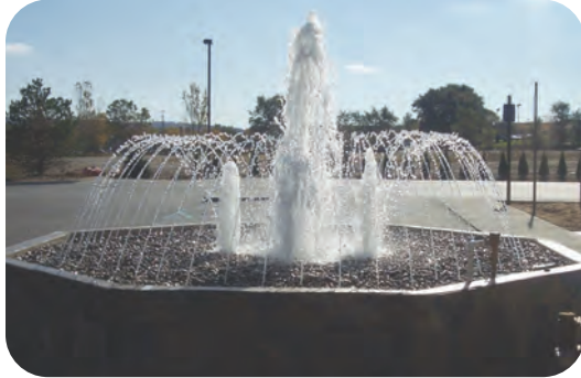
Nozzles can be installed vertically or at an angle. This feature has smooth jet nozzles surrounding frothy nozzles.
