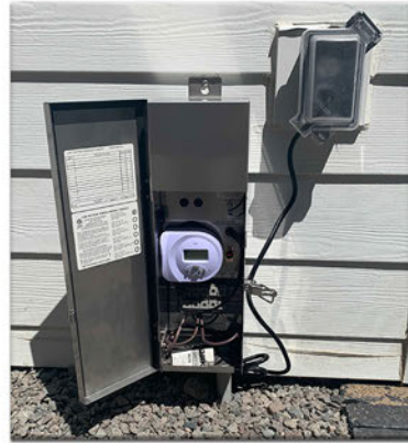
Plugs into any 120v GFI protected outlet shown with TRAT astronomical timer
